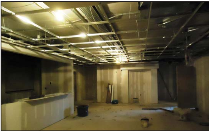
Interior is ready for drop ceiling.
