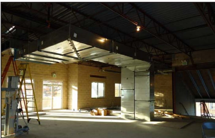
Mechanical work completed.
