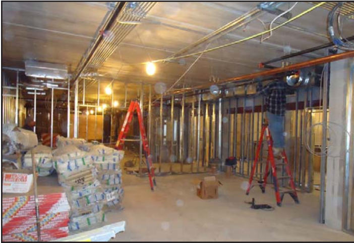
Mechanical work and rough-ins in the final stage.
