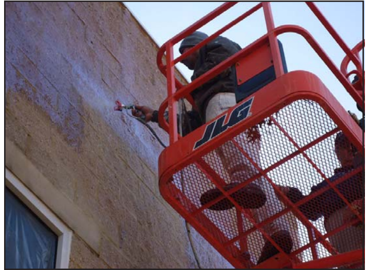
Volunteers from Superior and JNA Painting Co. waterproofing the exterior of the building.
