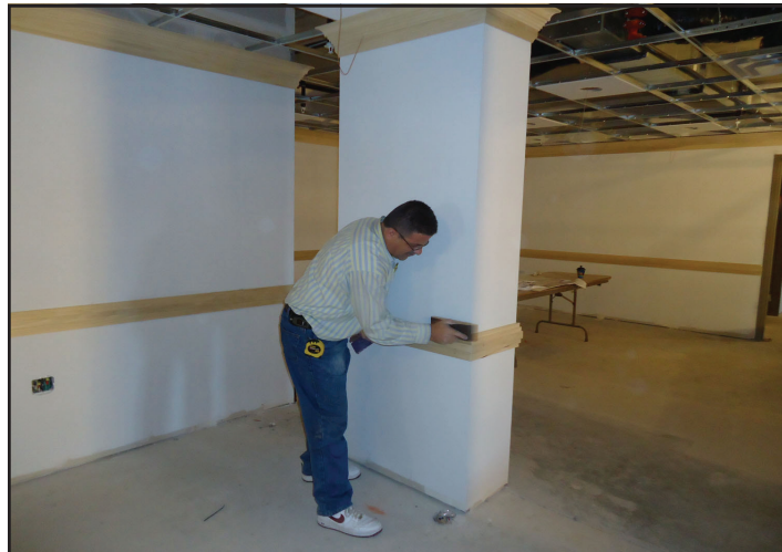
Decorative chair railing installed by ET Cabinets, Manolis Theoharis.
