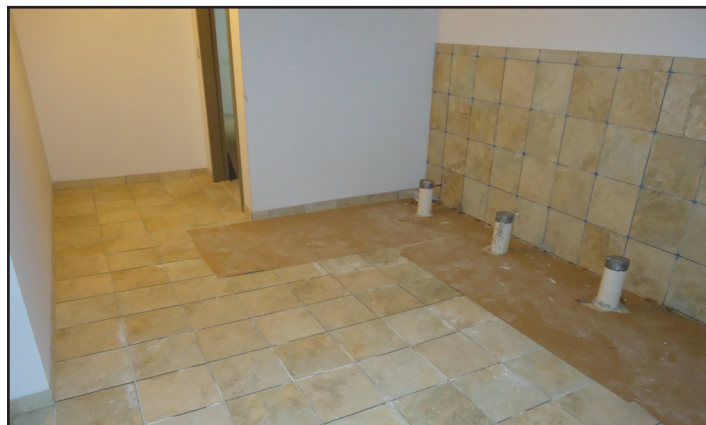
Ceramic tile laid on the bathroom floor and walls of the Plateia.
